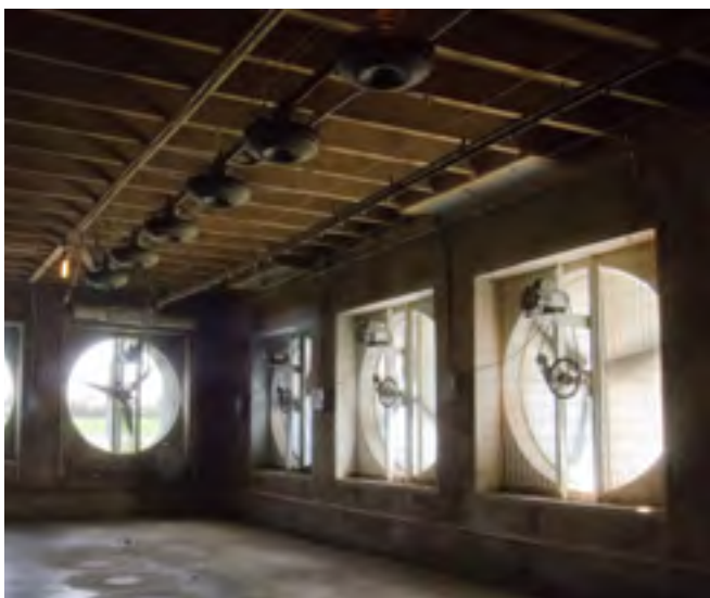
A mechanically ventilated chicken house relies on exhaust fans and automated inlets to regulate temperature, humidity, and air quality.
