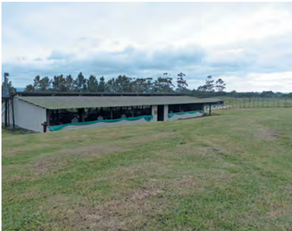
Some chicken houses use natural ventilation, like the house pictured above.
