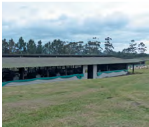
A naturally ventilated chicken house relies on wind pressure and warm air rising to exchange indoor air with fresh outside air.
